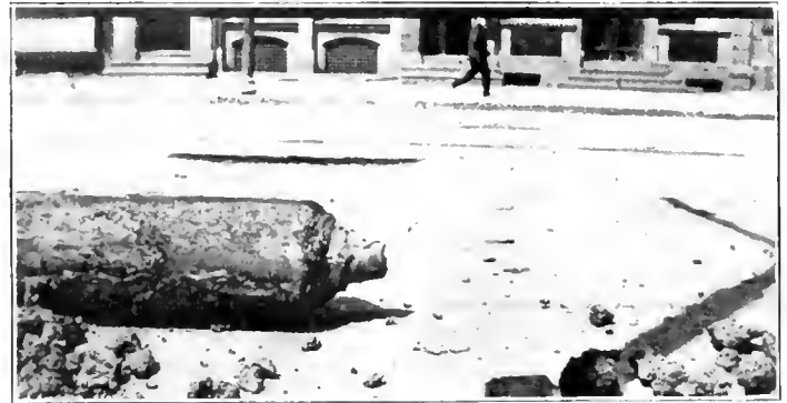
LOG WATER PIPE, BROADWAY, ALBANY, N. Y., LAID 1803—TAKEN UP APRIL, 1912.
